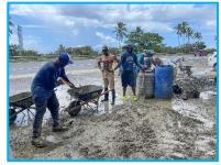
cement trucks getting flat tires on the way, we consistently received concrete that was already setting up, which made for poor quality material to pour our deck. Eventually we hired three local men who would mix the concrete all by hand on the ground. We would then transport it in wheelbarrows and bucket it up to our second floor.
